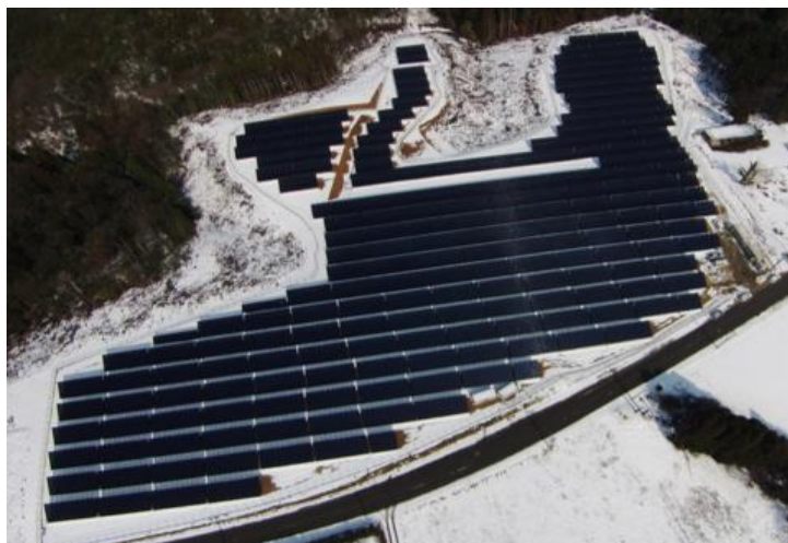
solar power generation facility owned by KLE
